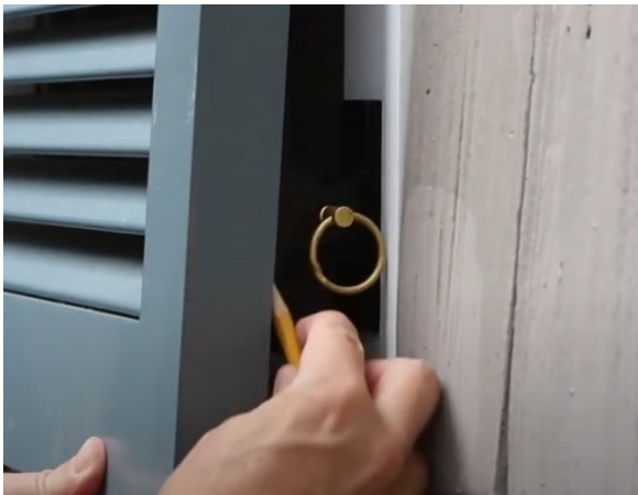
3.2 With a pencil mark the outer edge. Do it on both sides of the Panel.
