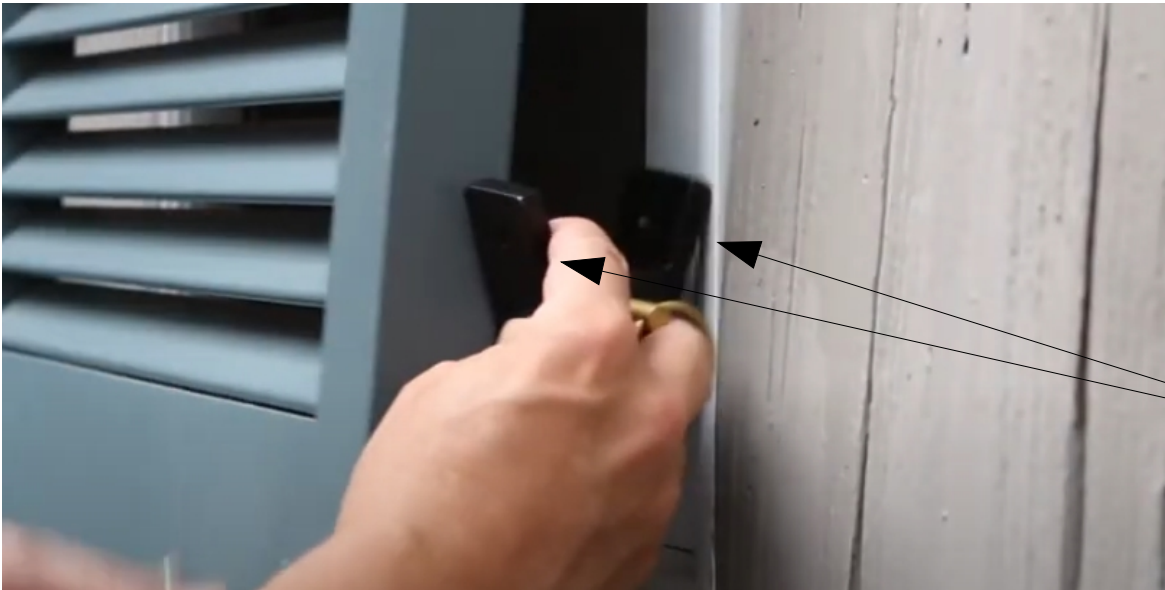
3.1 Hold the two brackets between the wall and with Shutter and mark the wall and the shutter
